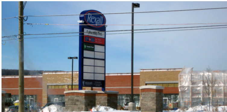
Fieldgate Commercial plaza under construction at Derry Rd. and Scott Blvd.
