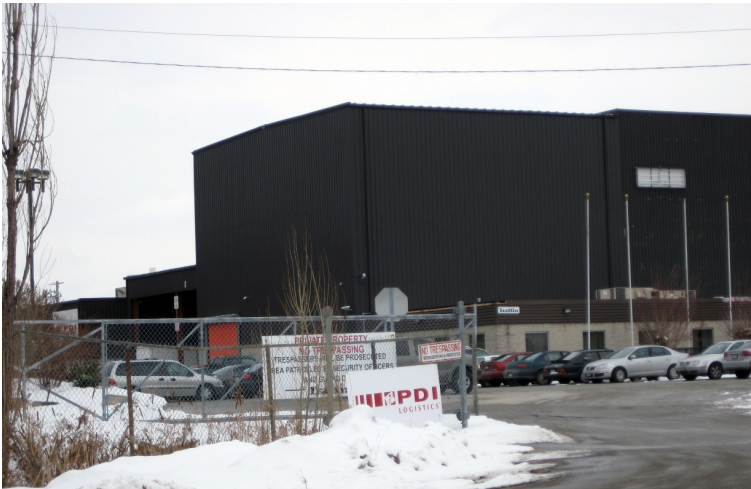
PDI Logistics facility at 375 Wheelabrator Way
